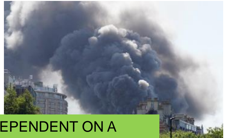
mandarin Oriental fire is believed to have been caused by the by-product of arc welding landing on the felt lining of the planting facade.
